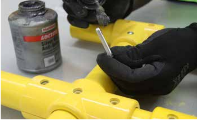
Anti-seize is applied onto each screw pre-installation
