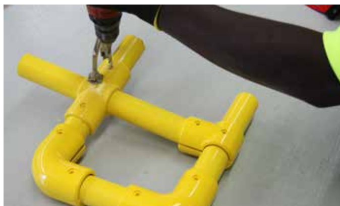
Holes are drilled
