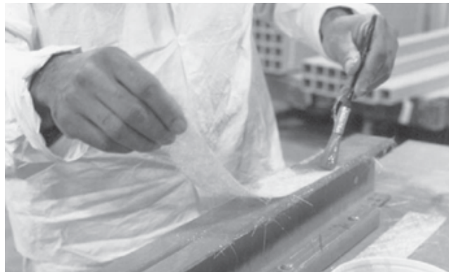
Joint taping with fiberglass mat and resin.
